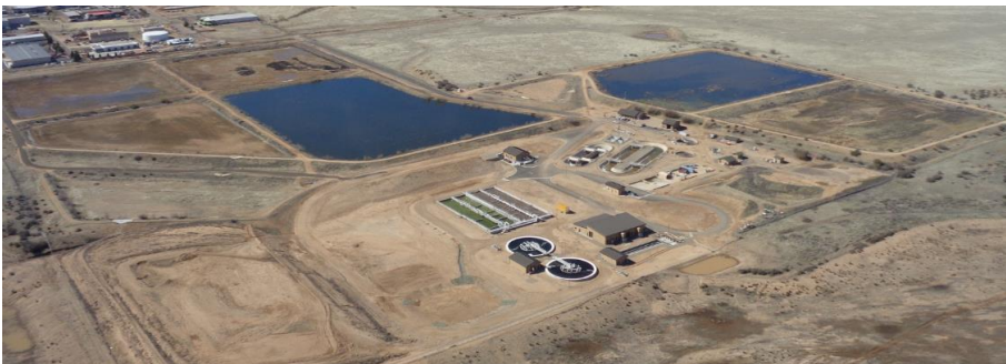
City Recharge Facility
